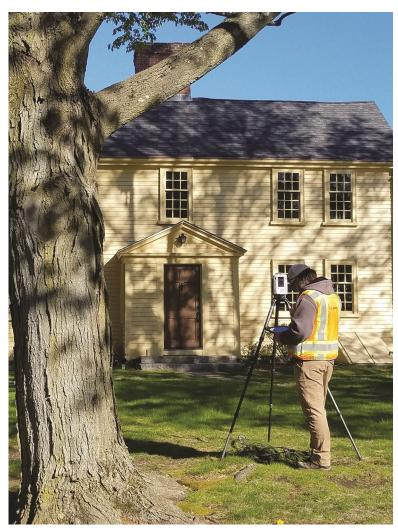
Technicians from Feldman Surveyors conducted a laser scan of the Jason Russell House and grounds May 14 and 15, 2020. A limited crew size enabled working within physical distancing guidelines. The data revealed will provide incredibly technical documentation of the current conditions of the house.
